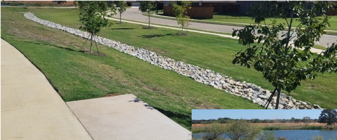
In progress - Rip Rap/Drainage Project
